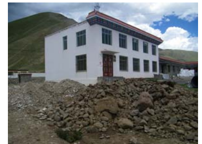
View of recent building that will have to be rebuilt
