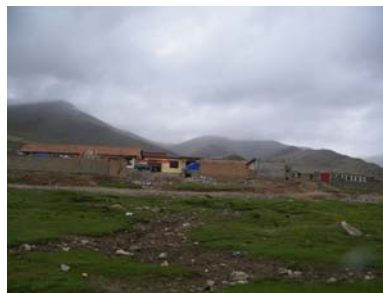
View of entry to clinic site
